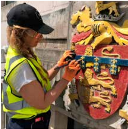
Student stonemasons restoring the Duchy crest at Lancaster Place.
