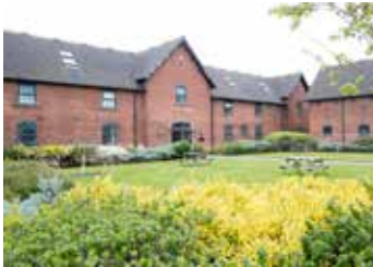
Crewe Hall Farm offices, Crewe Estate, Cheshire.
