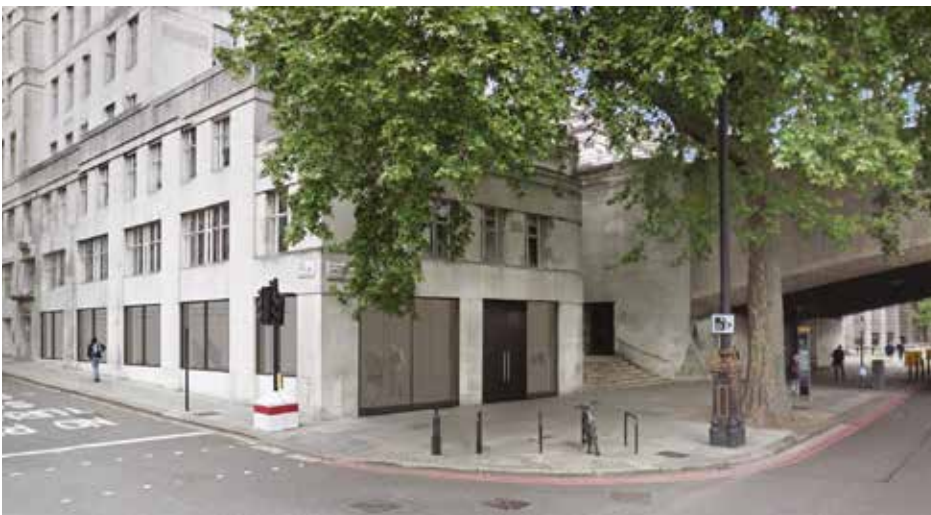
Refurbished ground floor offices, 9 Savoy Street, London.
