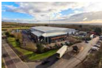
Ravensbrook Business Park, Redditch.
